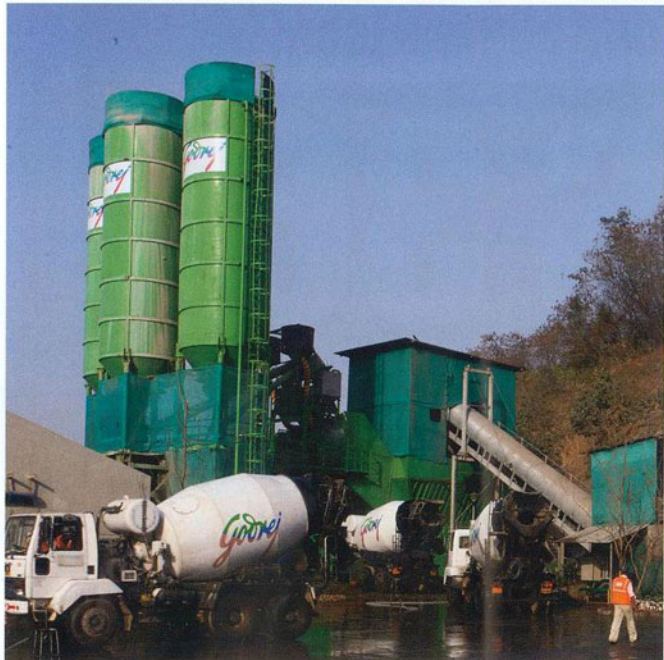
Godrej Construction uses automated batching plants extensively for its operations.
